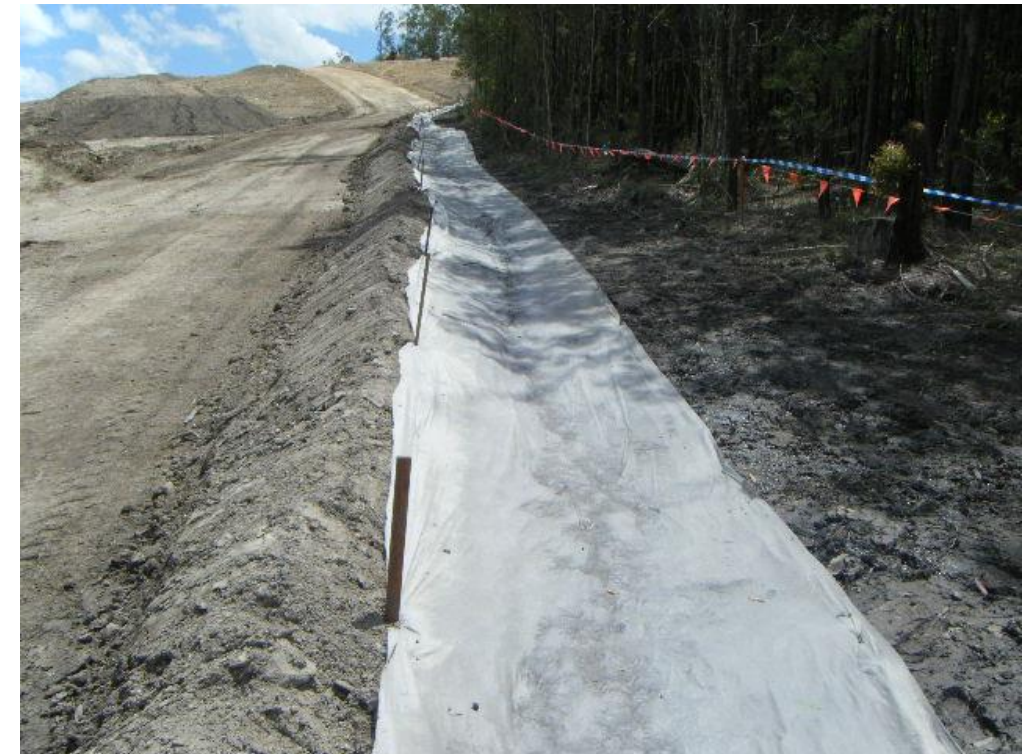
Stage 2 - The topsoil spillway area has been covered with pinned geotextile with plastic underlay, and scour rock.
