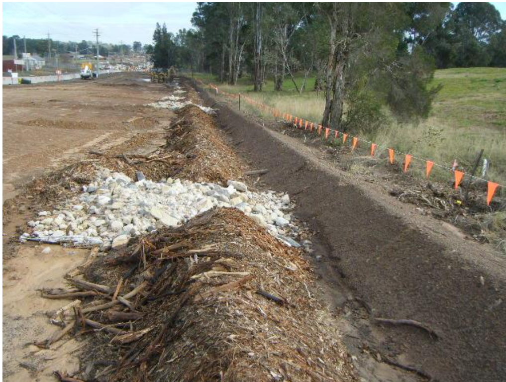
Stage 1 - Topsoil formed in a compacted formation with spillway cut.
