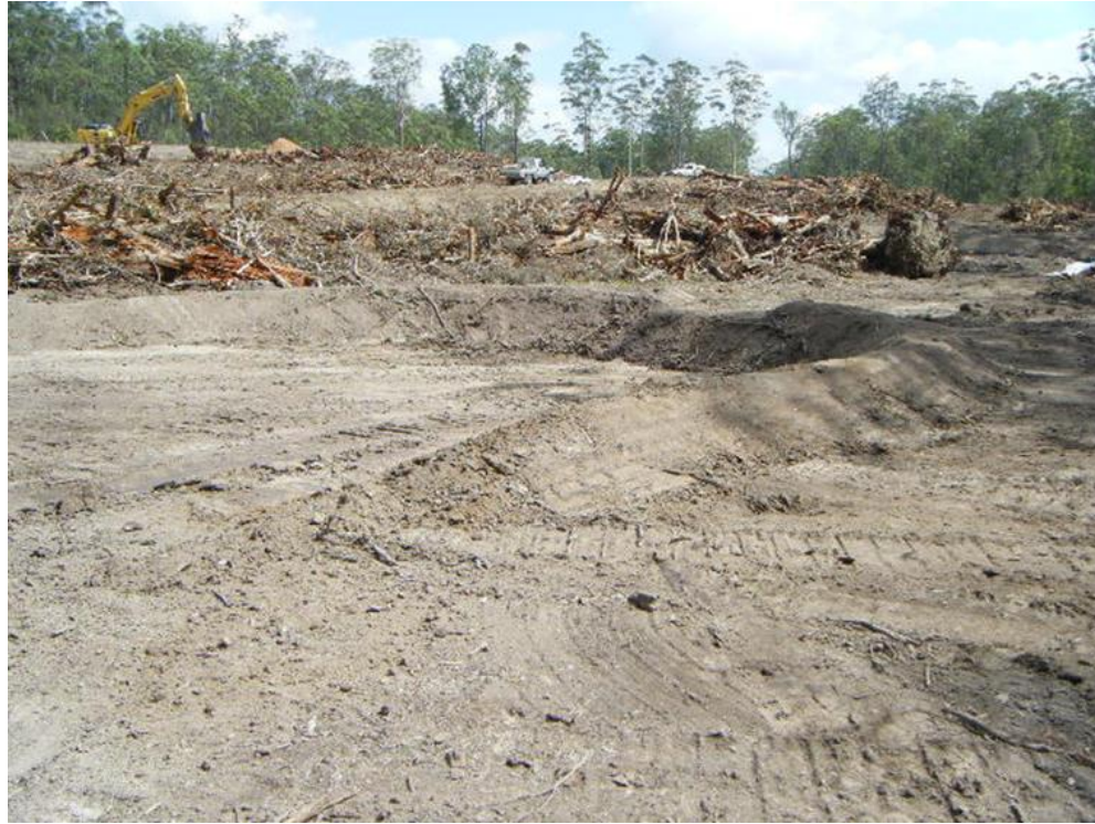
Stage 1 - Topsoil formed in a compacted formation with spillway cut.
