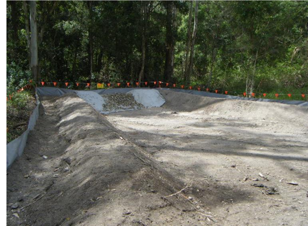
Stage 2 - The topsoil spillway area has been covered with pinned geotextile with plastic underlay, and scour rock.
