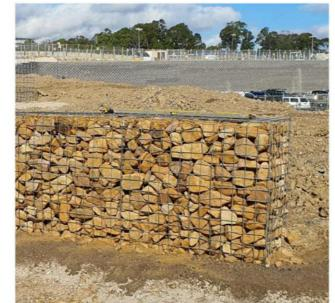
Rigid stainless steel gabion cage with 75-150mm sandstone spall
