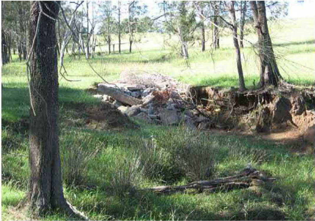
Concrete blocks downstream of former rubbish disposal area.
