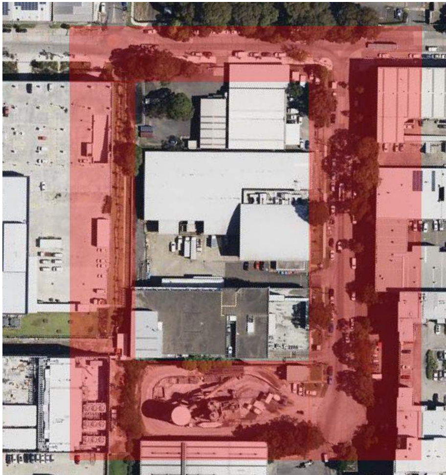
Image 1 – Proposed development and inspected buildings and infrastructure (external inspection only)
